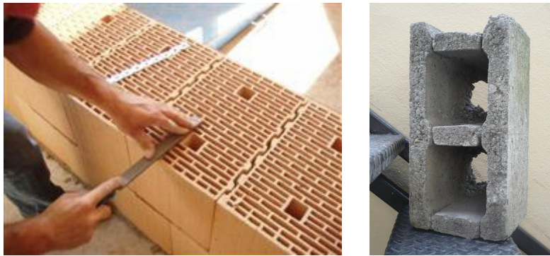
Figure 8: 'Thermoplan Ziegel' wall from NBT and an Irish hollow block
